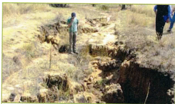
Figure 1. Tunnel and gully erosion resulting from construction of a stormwater culvert in dispersive clay.
