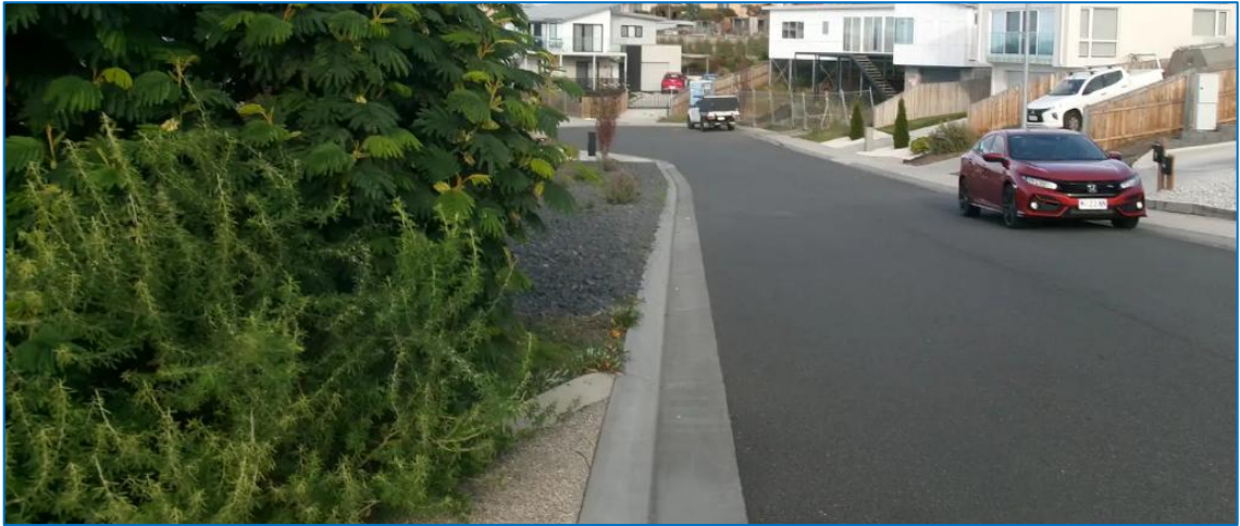
Photograph 7.2A – Available sight distance to the left (when vegetation is removed)
