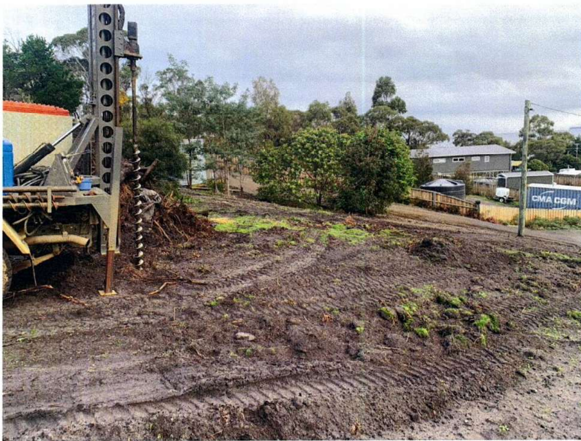
Plate 2 – Lot 1. Test Hole #2 - Looking to the southeast.
