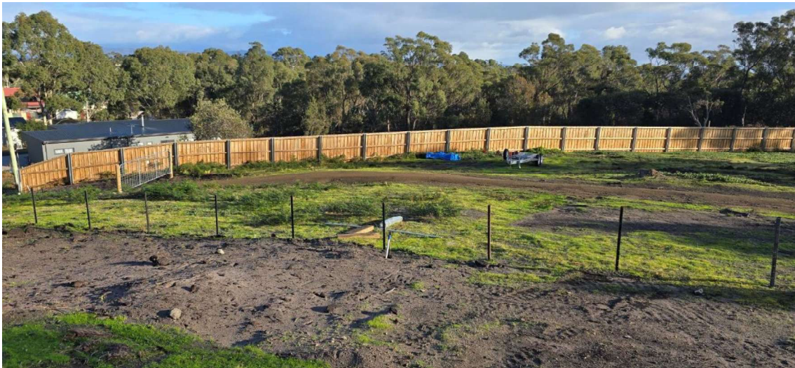
View of current condition of block to the north
