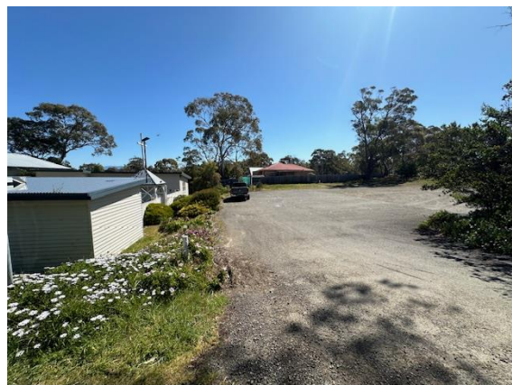
Figure 14 sealed access to ROW and car park
