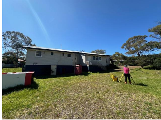
Figure 12 Main Hall south elevation
