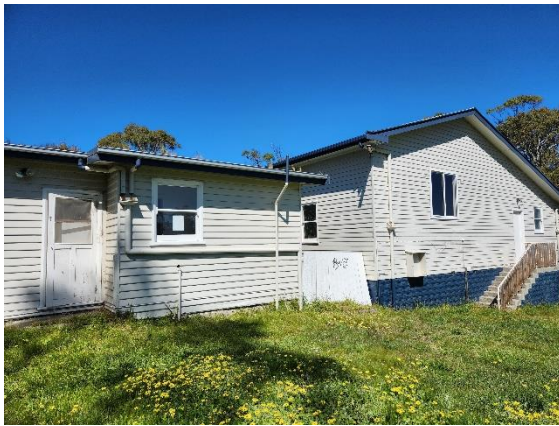
Figure 7 Main Hall and secondary hall A looking SE
