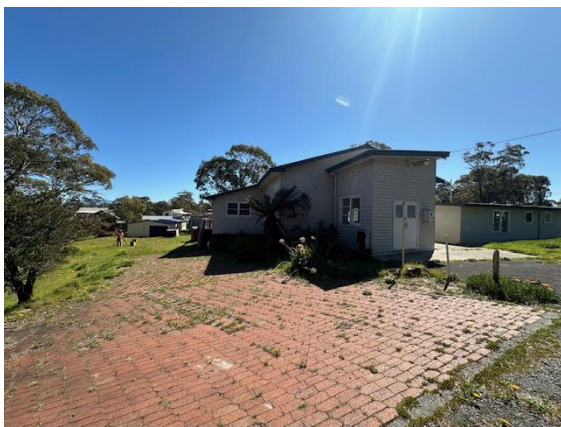
Figure 13 Paved access from ROW
