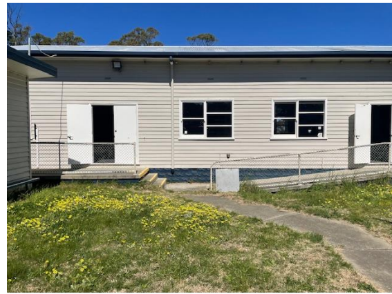
Figure 8 Main Hall looking South
