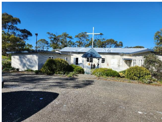
Figure 3 View from car park to three halls - looking south
