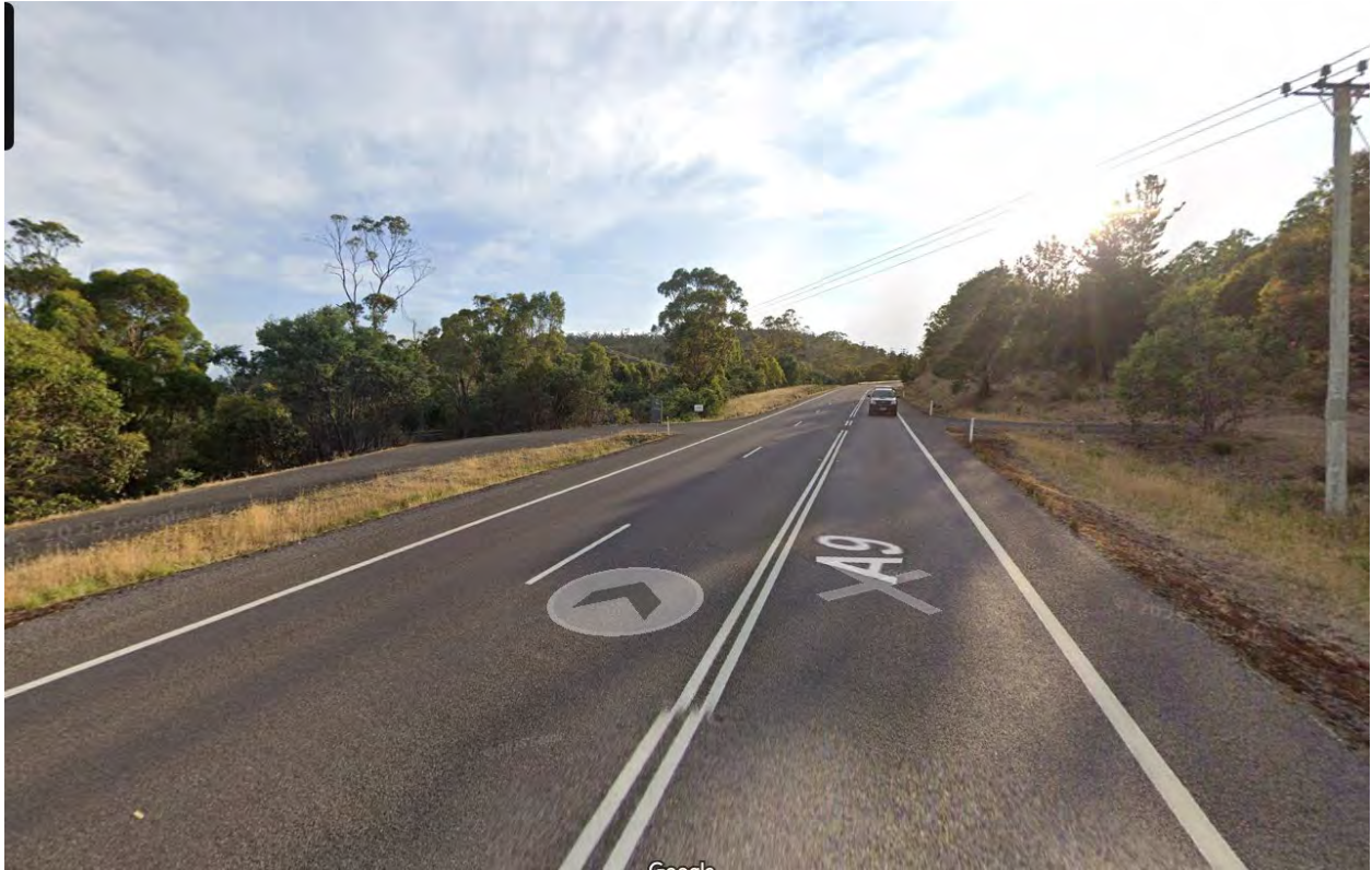
Figure 4. Intersection (facing east).
