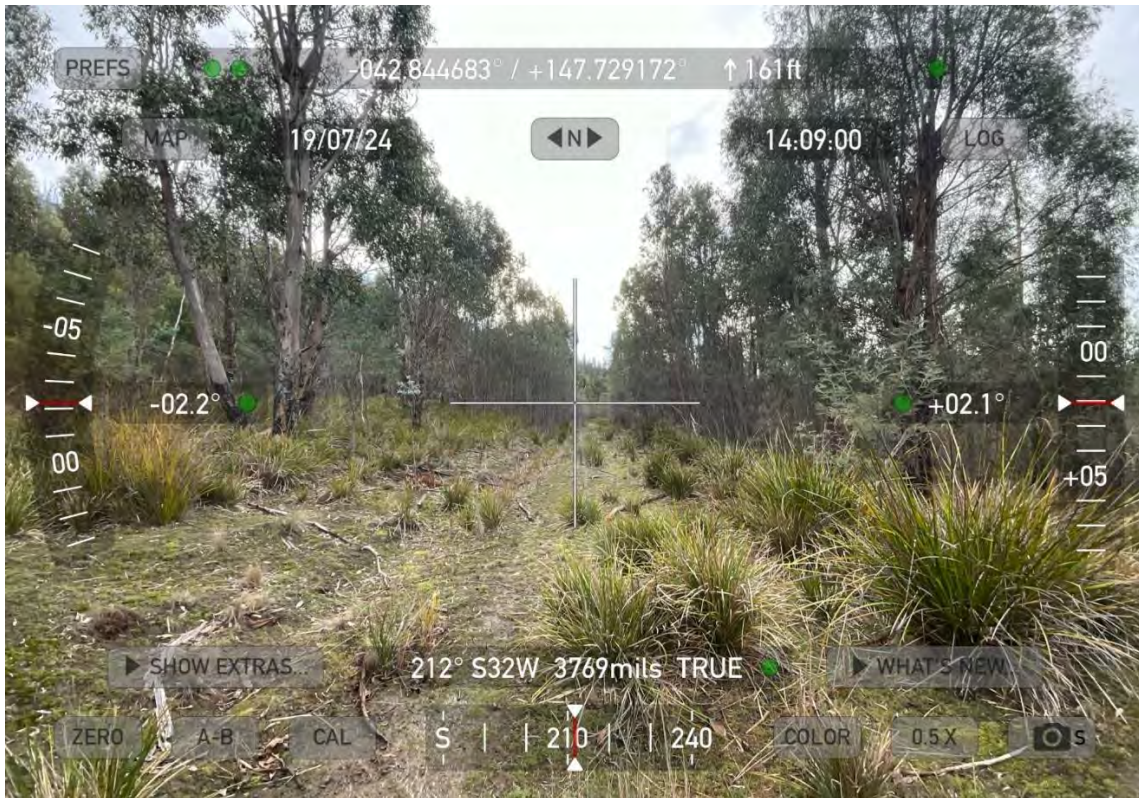
Photo 1 - Road section between lot 10 and 13
