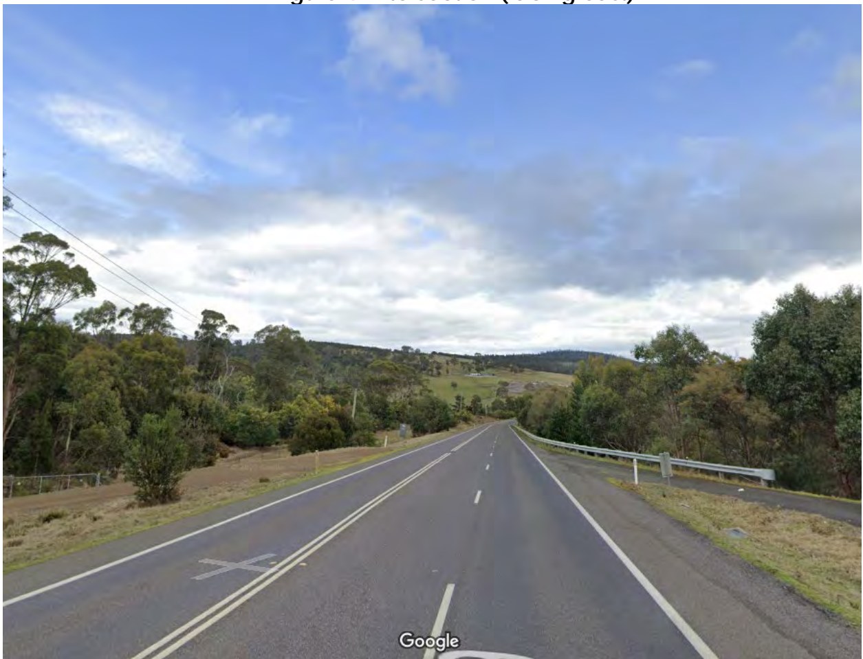
Figure 5. Intersection (facing west).
