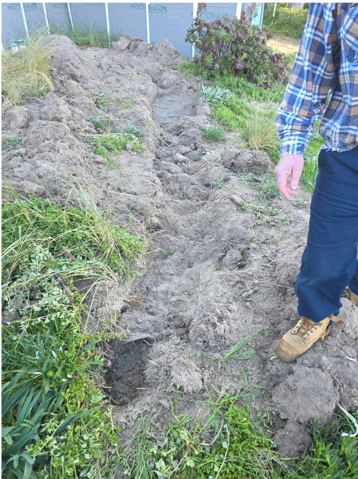
Figure 2: Exposed existing wastewater treatment trench
