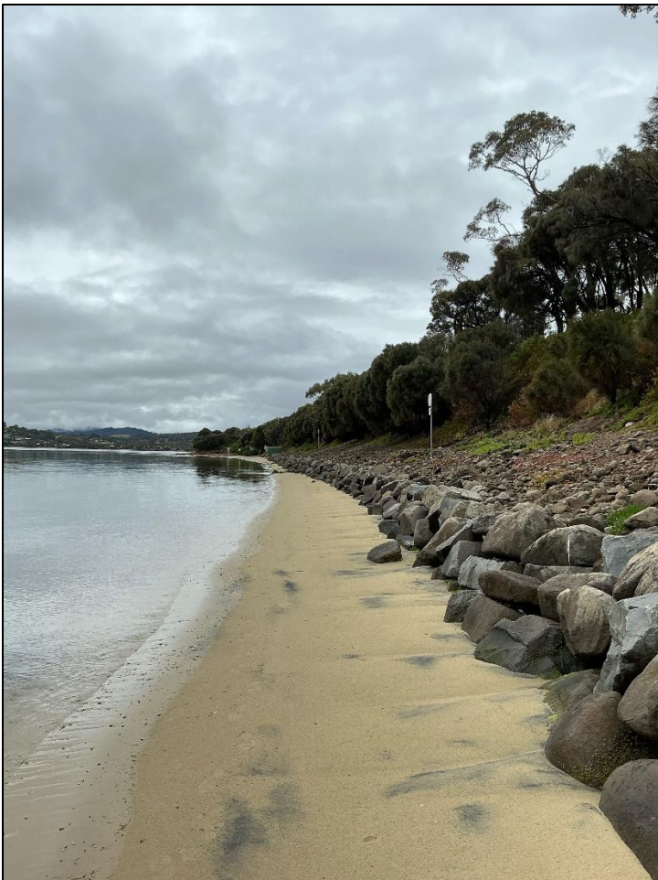
Photo #4 Coastal protection works along the beach made from dolerite boulders. The steep slope is clearly visible as well. The mean high water mark is at the coastal protection works
