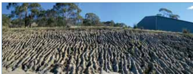
Figure 17. Extensive 'outlet initiated' tunnel and rill erosion caused by excavating a cut and fill pad for a large building in a dispersive soil. Triassic sandstone parent material.
