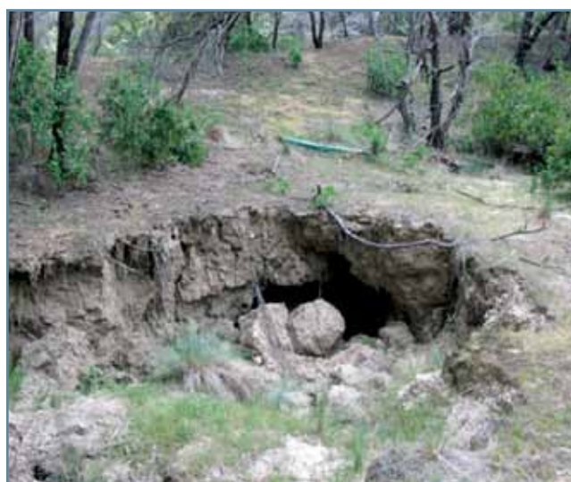
Figure 34. Piping failure of a dam constructed from soils derived from Permian mudstone, Penna area. This dam is known to have failed on first filling. The image was taken from the dam floor, looking at the inside of the dam wall.
