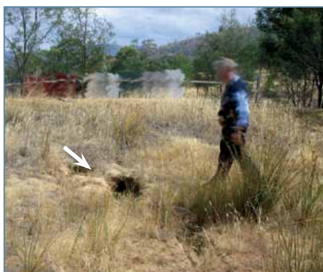
Figure 33. Typical small dam failure. Note piping through the side wall of the dam. This dam was constructed using dispersive clays derived from Triassic sandstone.
