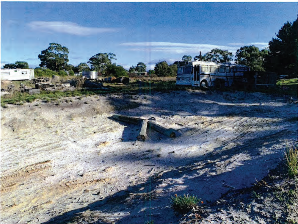
Plate 2 Deep sand exposed in the partially excavated driveway access cutting.
