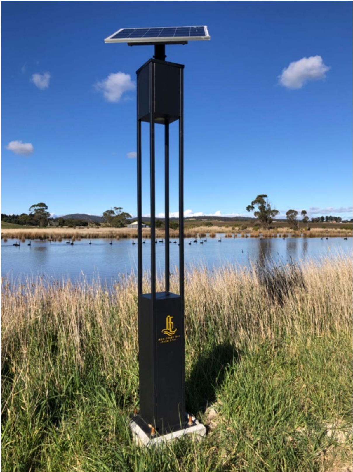
Solar lights – 3m high including an internal downlight sited 2.1m above ground
