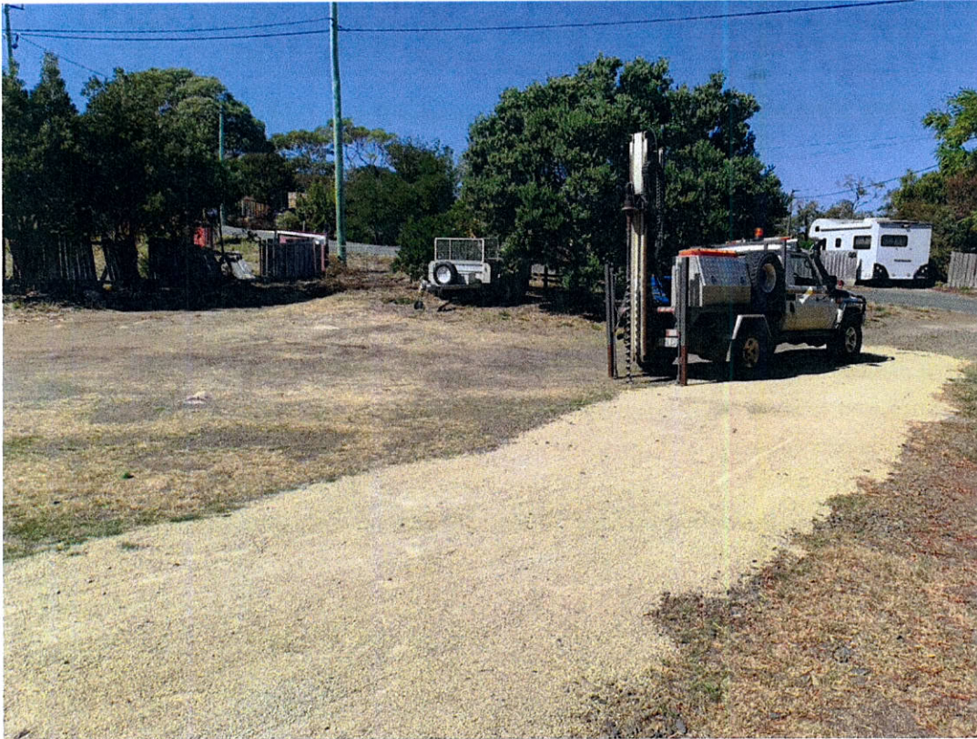
Plate 2 – Test Hole #4 - Looking to the south / southeast.
