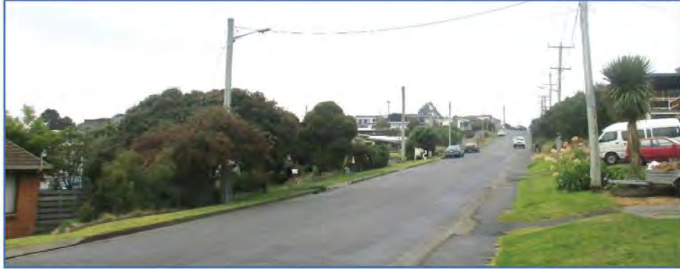
Photograph 7.5A– Available sight distance for a driver looking right when leaving the site
