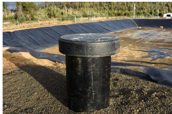
SS14: Secondary SWP – Seepage Pit
