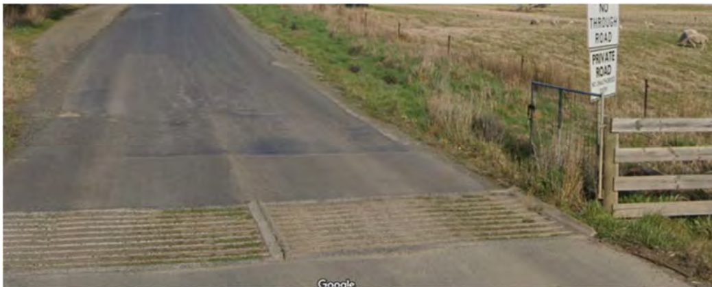
Photograph 1: Showing the sealed section of Blue Hills Road.
