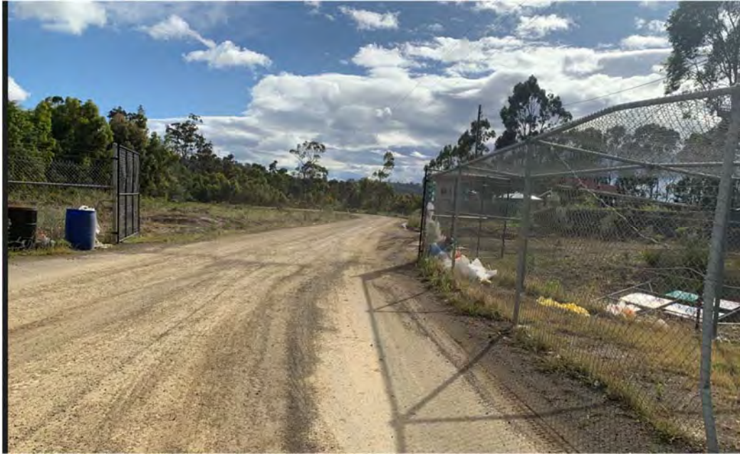
Photograph 2: Showing the gravelled road access to the Southern Waste Solutions site which is ~ 7.5metres wide.
