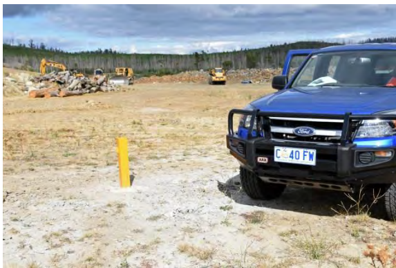
BH23: B-Cell Near Cell 7-14 Bore
