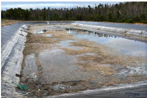
SS9: C-Cell Leachate Balancing Pond
