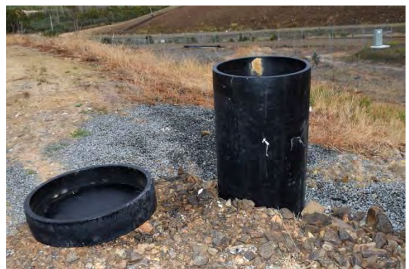
SS11: C-Cell MLP-Seepage Pit
