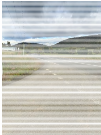
Photograph 5: Sight Distance at the intersection of the Arthur Highway and Blue Hills Road was measured to the right (west) metres to be in excess of 200-metres.
