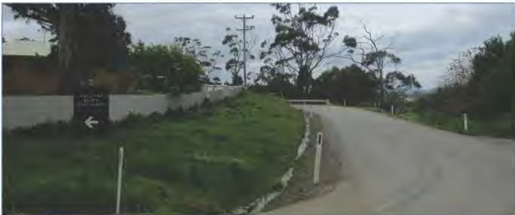
Photograph 9.0D – Possible benching of embankment to increase sight distance
