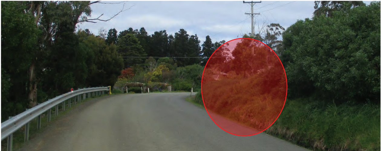
Photograph 9.0D – Possible benching of embankment to increase sight distance
