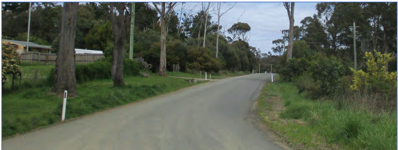
Photograph 9.0C – Available sight distance for motorists looking right (exceeds 150 metres)
