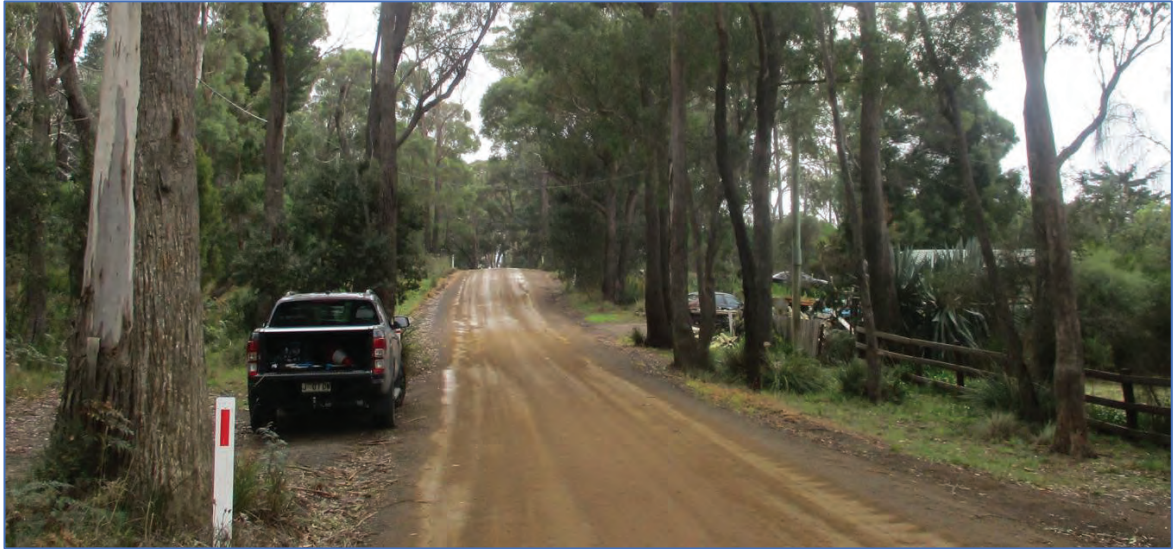
Photograph 6.1B – Typical Road standard of Craigs Hills Road (section two where trees reduce the trafficable road width to less than 5.5 metres)
