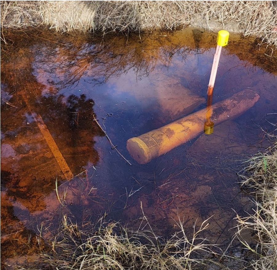
Figure 6: Temporary outlet from Blue Lagoon operational during peak rainfall
