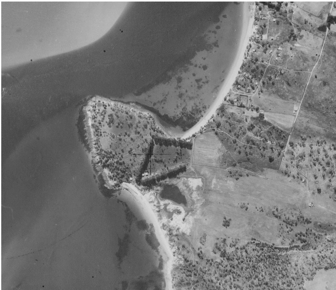
Figure 3: Historical image of Dodge's Ferry area taken on 8 April 1949 (Photo source: DNRE)
