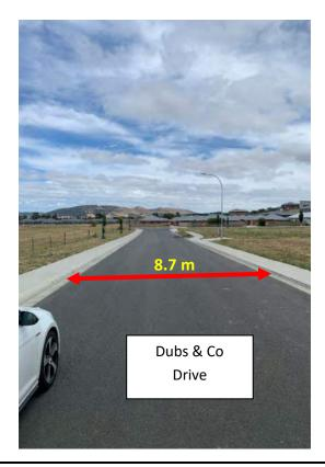
Photograph 4: Road width is 8.7-metres measured between kerb faces.
