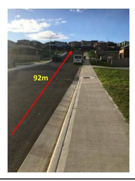
Photograph 6: Sight Distance at the exit was measured to be 92-metres towards the north.
